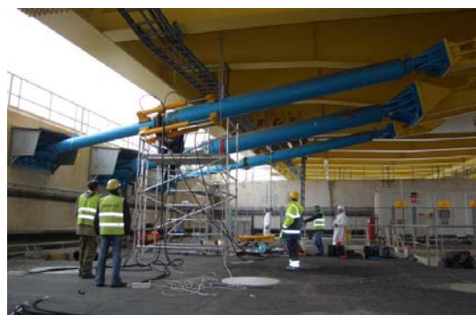
Fig. 18 Deck re-alignment & preparation for fuse replacement at pylons
